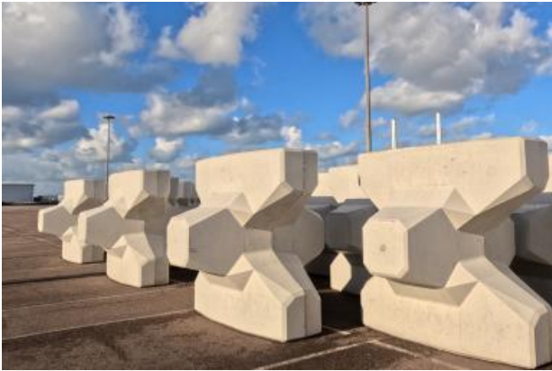
construction, development Production of Accropodes™ for the « chatière » breakwater is underway
