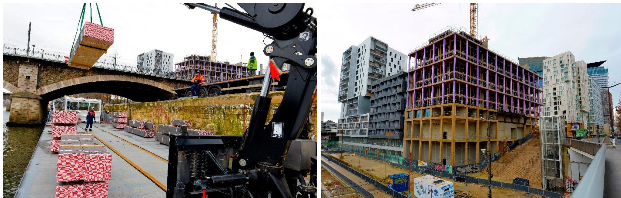
Caption: transfer by SOGESTRAN LOGISTICS's Zulu barge of wood components for the Wood Up tower under construction in Tolbiac. Credit: © HAROPA PORT – Nautilus. HR pictures on this link
